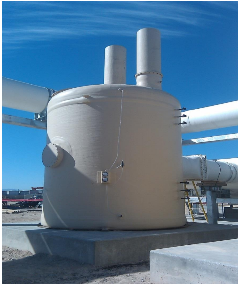
Figure 19. Solids Handling Adsorber SHF-2B #5 Carbon Adsorber Facing North
