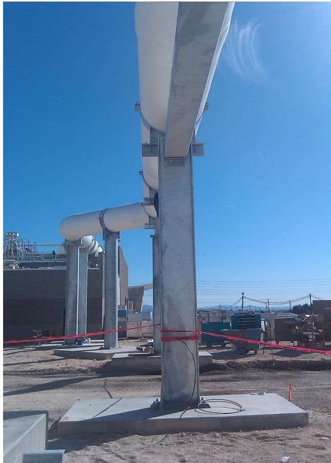
Figure 3. Typical Section of the Odor Control System Ductwork Facing North
