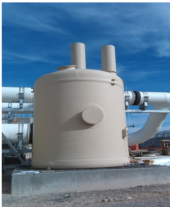
Figure 1. Typical Carbon Adsorber Vessel Facing North
